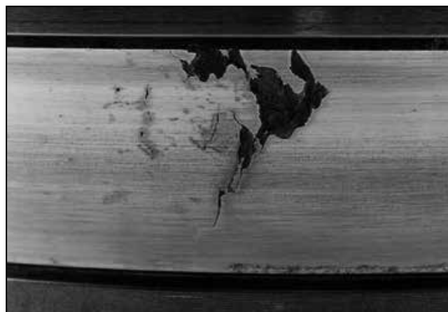
Fig. 170. Point surface origin spalling (PSO).
