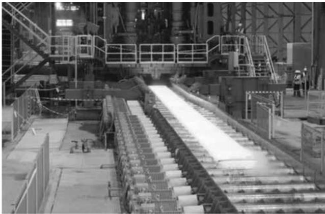
Fig. 113. Hot-strip mill transfer roller table.
